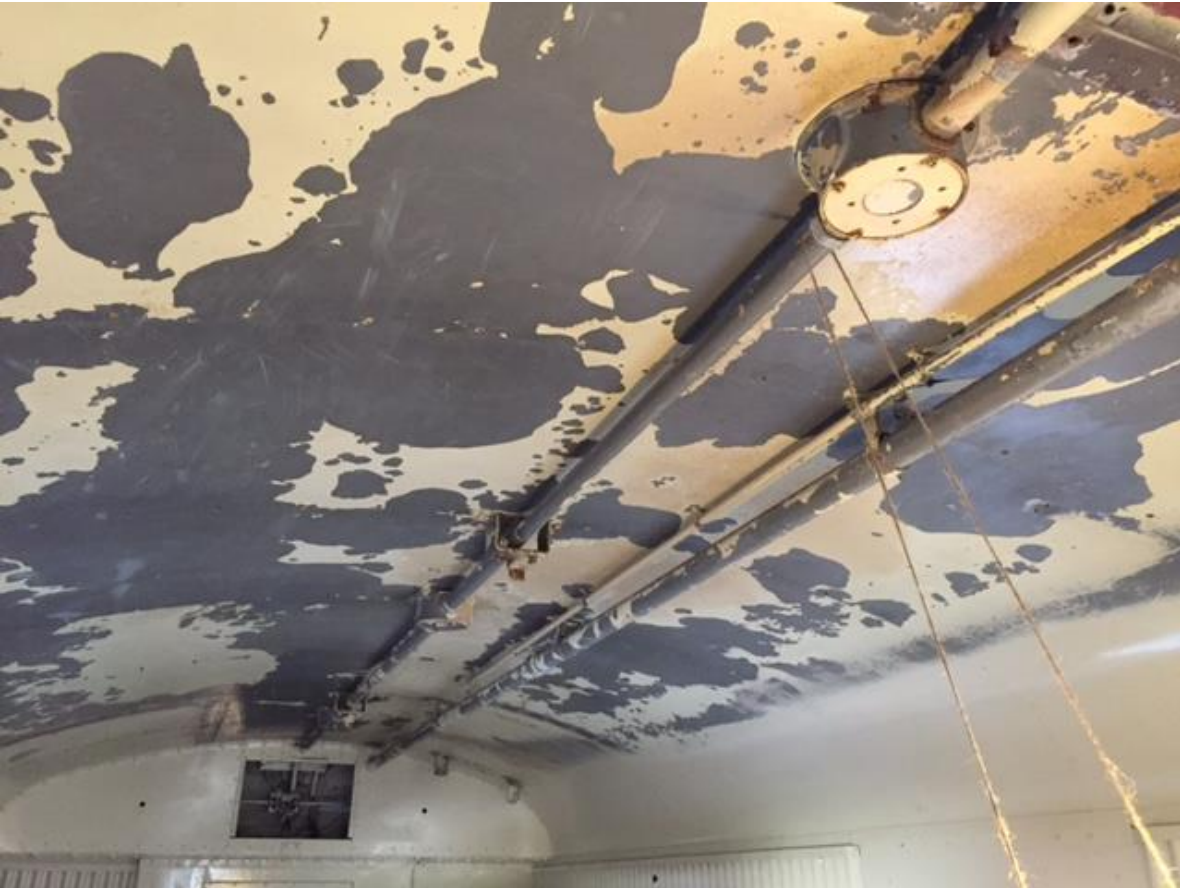
A view of the inside of UP5642 before the restoration
