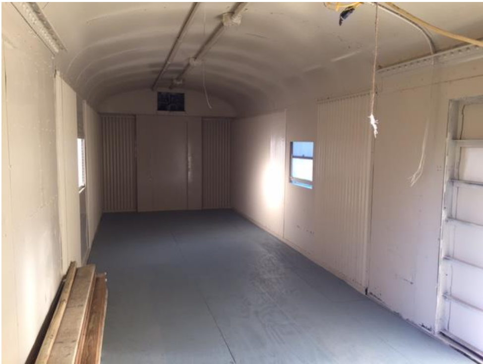
A view of the inside of UP5642 during the restoration
