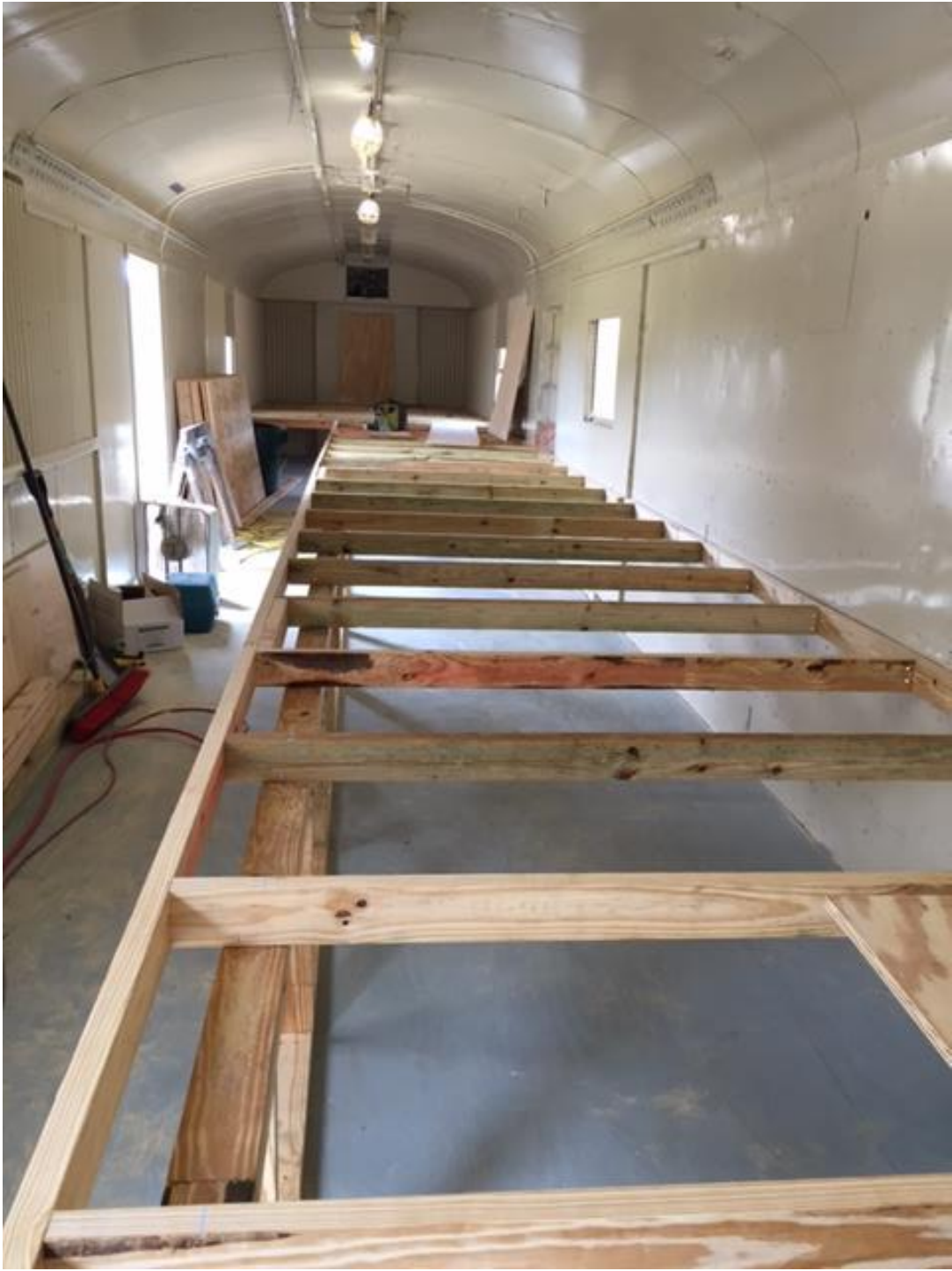
Starting to lay out the bench work for the G-Scale layout
